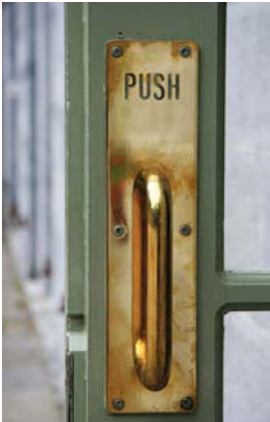
FIGURE 7.2 This door handle reads PUSH but its design encourages you to pull
